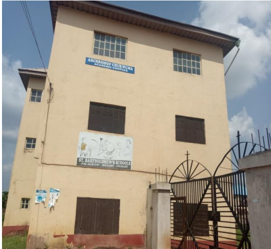
Fig 1: St. Bartholomew's Primary School Building
