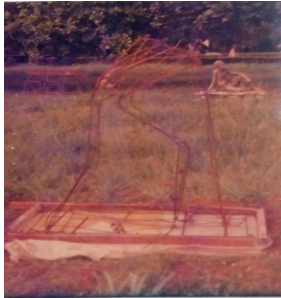
Plate 2: Base Construction by Ogba, O. M.
