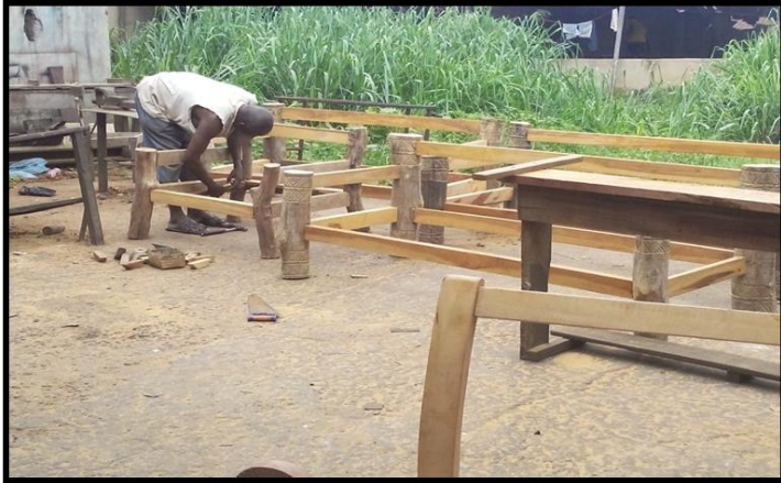
Plate 15 : Work in progress
