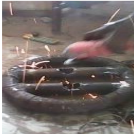
Plate 11: Welding of parts
