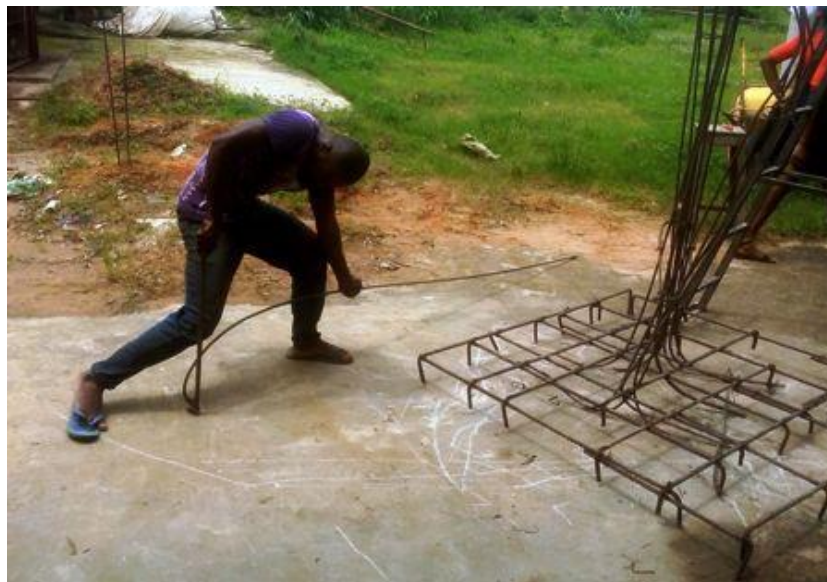
Plates 7: Armature construction. Source: the sculptor
