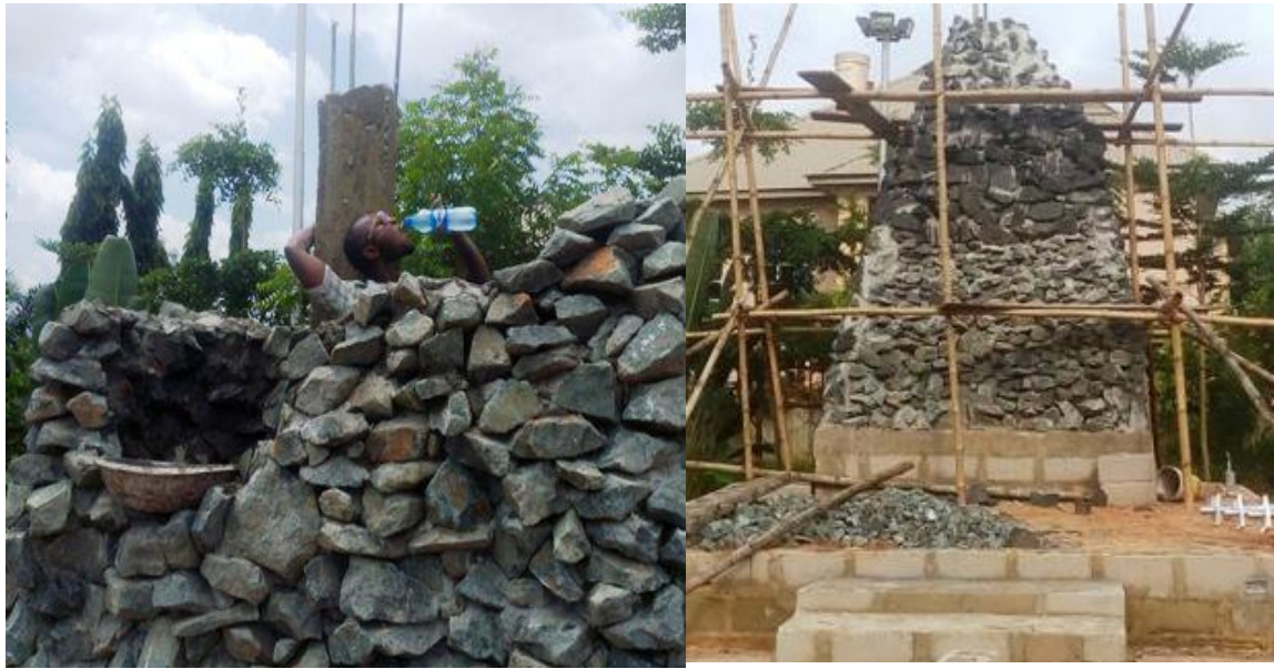
Plates 16-17: Showing different stages in the building of the stone pyramid for the Grotto of Christ Crucified. Source; the sculptor.
