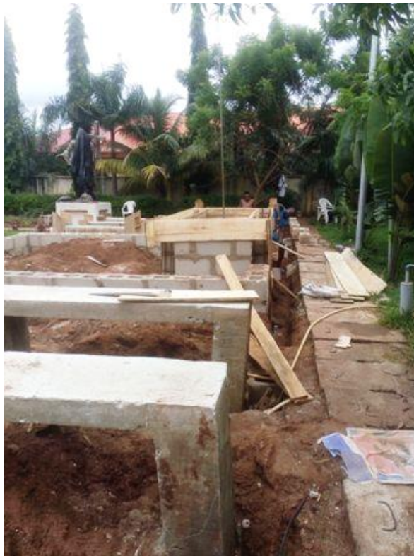
Plate 14: Initial concrete structural base for the Grotto. Source; the sculptor
