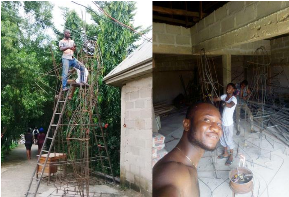
Plates 5 and 6: Armature construction. Source: the sculptor
