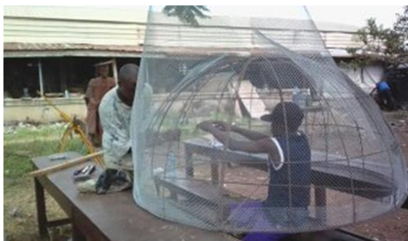
Plate 7: Covering the Armature of Globe with Galvanized Wire Mesh © The researcher, 2018
