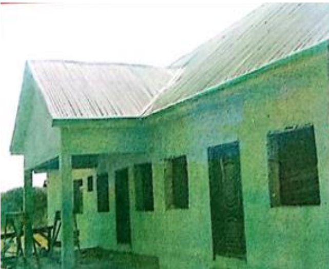
Fig 5: About to be completed IMAN Secretariat, Bida
