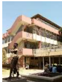
Plate XIII: Cantilevered Staircase, Department of Architecture, ABU Photo: Authors 2020
